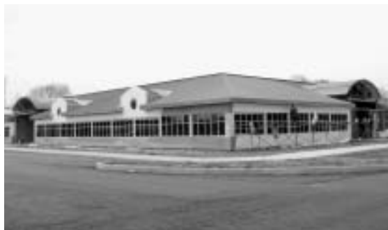
Palisades Medical Center in West Nyack
